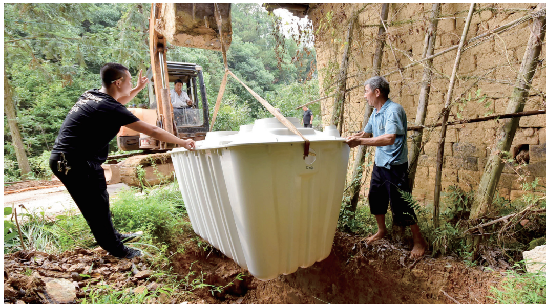
Workers help villagers install underground storage tanks for a sanitary toilet in a remote village in Hunan Province, Aug. 25, 2021. Photo: CFP
