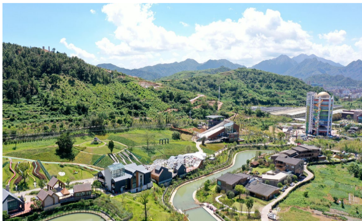
A demonstration village in Wenzhou City, Zhejiang Province Photo: CFP
