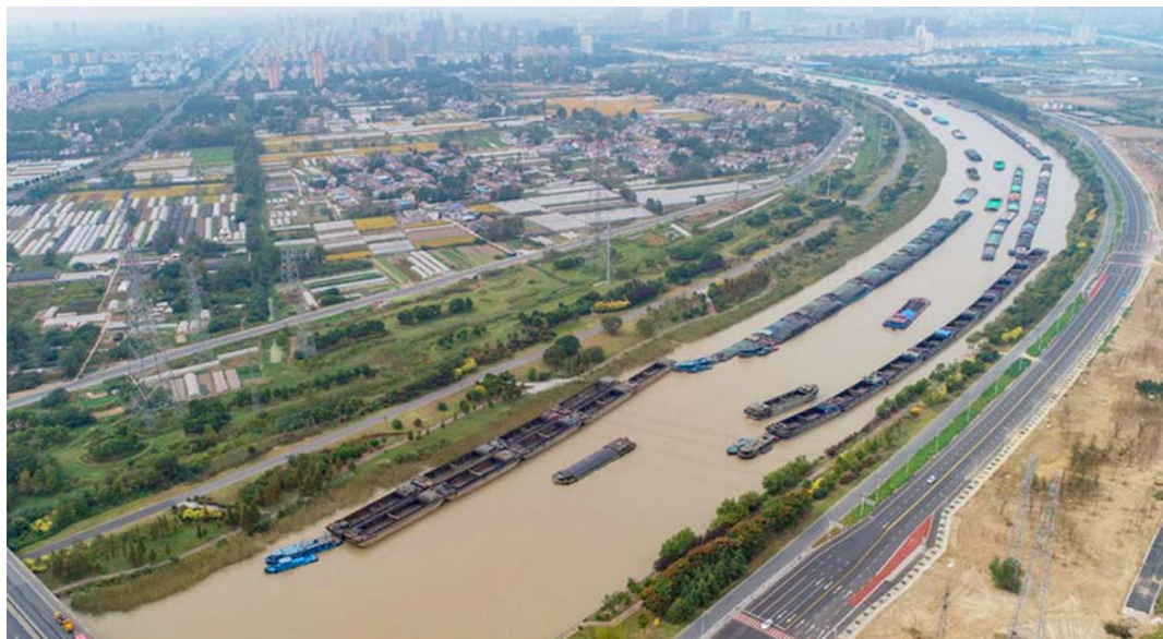
Barges navigate a section of the Grand Canal in Huaian City, Jiangsu Province. Photo: CHINA DAILY
